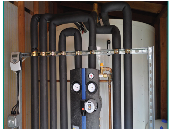
Haase Energy solar storage tanks are un-pressurized fiberglass reinforced plastic. Modern materials eliminate rust and corrosion problems common with steel tanks, and extend the life of the system.
